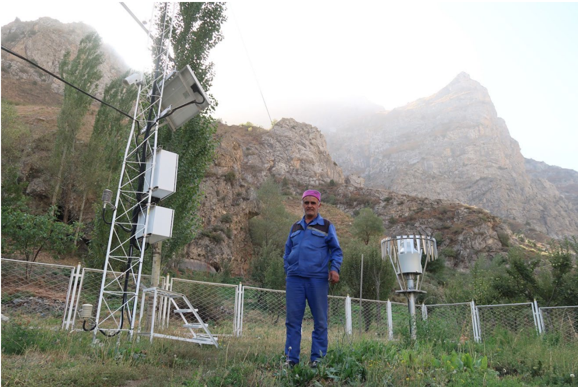
Figure 7. Modern automatic Snow station (left) in Tajikistan under the World Bank financed the Central Asia Hydrometeorology Modernization Project (CAHMP) project, equipped with modern snow depth laser (Lufft), together with a pluviometer (right) and snow measurement stake (centre).
